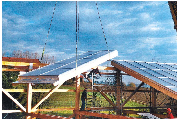
Figure 21: Crain assembly of the entire roof elements with support construction and collector field (picture source: Wagner & Co, Germany).
