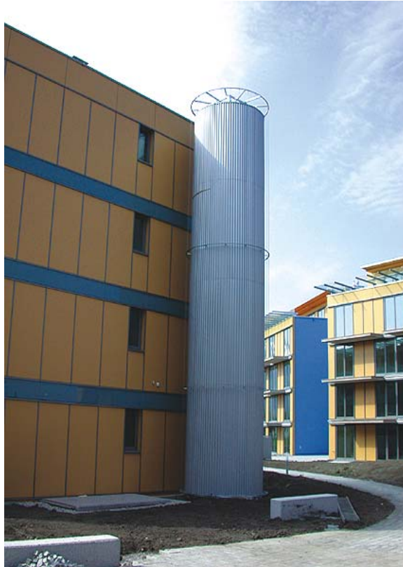
Figure 44: Energy storage tank integrated deliberately visible in the building (picture source: AEE INTEC).
