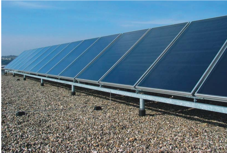
Figure 29: Large-area collectors mounted with a continuous construction. The construction is fixed on the roof on only a few places and the breakthroughs to the roof can thereby be reduced discontinuity (picture source: AKS DOMA Solartechnik, Vorarlberg, Austria).
