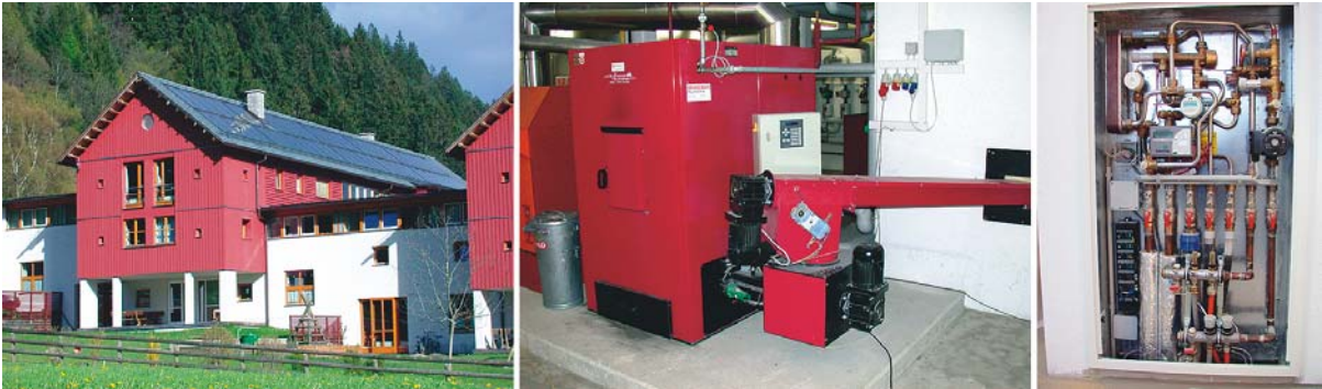
Figure 4: Efficient solar-supported heating networks demand a holistic approach to the planning, implementation and management. This includes the solar thermal system (left), the conventional heating systems (middle, in this case biomass) as well as the heat distribution system (right) (picture source: AEE INTEC).
