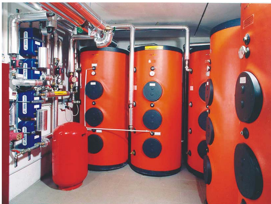
Figure 101: Multi-storage-unit systems result in heat losses, not only in solar thermal applications, but also in conventional heating systems (picture source: AEE INTEC).
