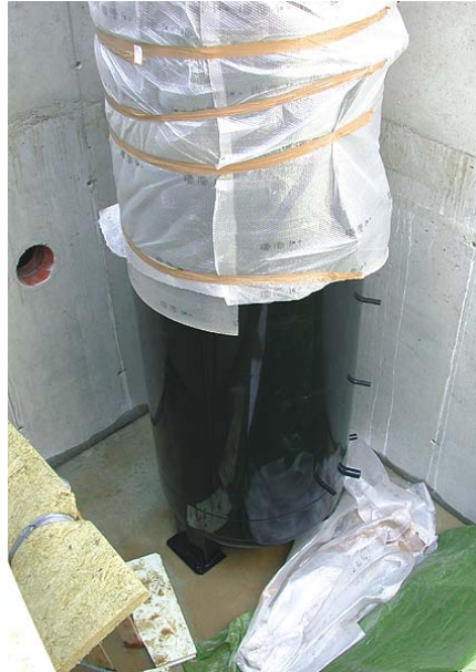
Figure 43: The energy storage tank is as standard lowered into the foundation and installed prior to the construction of the basement ceiling (picture source: AEE INTEC).
