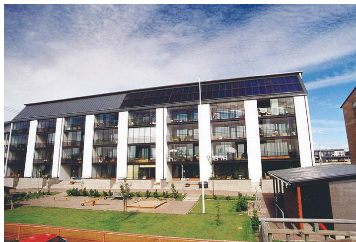
Figure 2: 1.248 m 2 solar thermal collector area produced by an Austrian manufacturer on the roof of eight multi-storey residential buildings in Helsinki (picture source: AEE INTEC).
