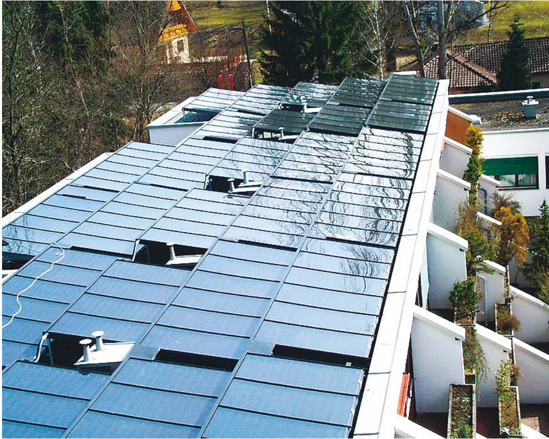
Figure 84: Solar-supported heat supply system for the housing estate "Hans-Riehlgasse", erected on the existing building. The solar thermal system was connected to a four-pipe network, since this was already at hand (picture source: S.O.L.I.D.).
