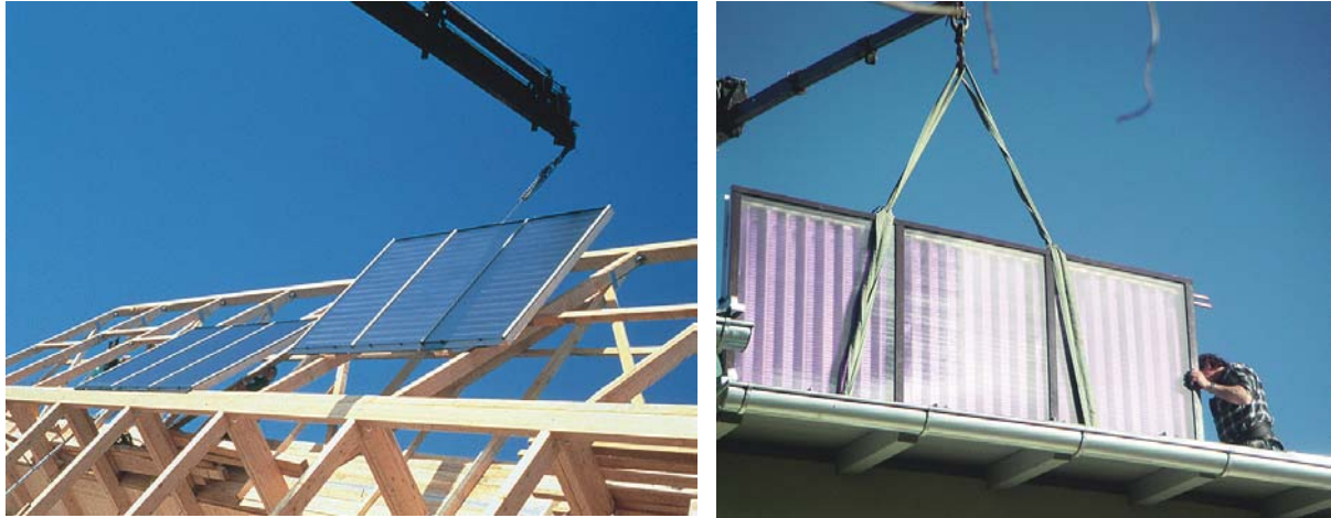
Figure 50: Standard by the solar thermal systems in multi-storey residential buildings: crane mounting of the large area collectors (picture source: AEE INTEC (left), SIKO Energiesysteme, Tyrol, Austria (right)).
