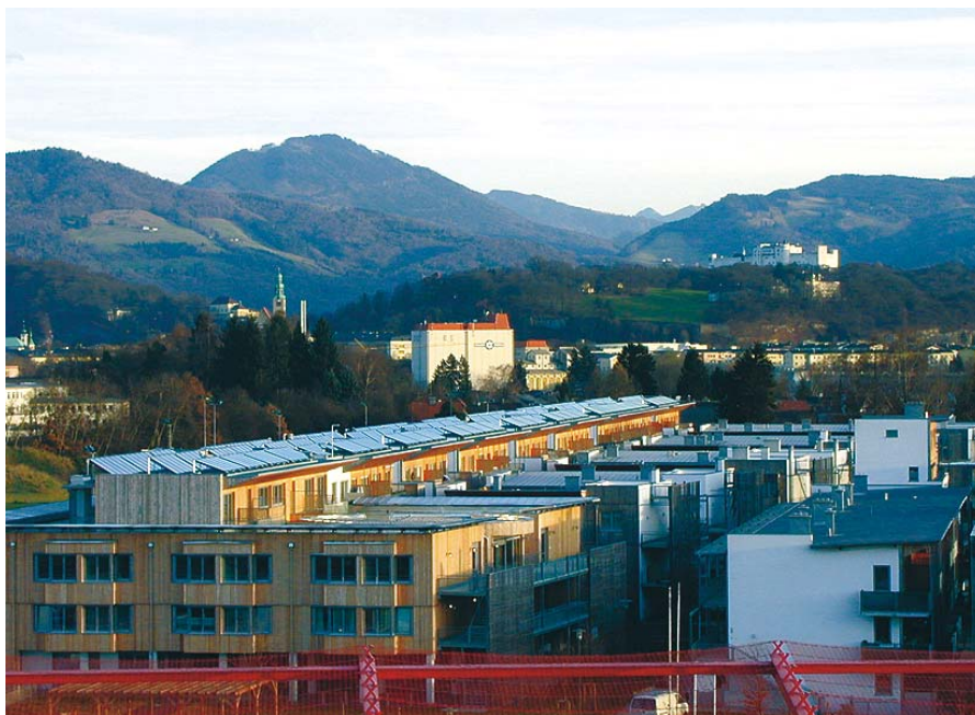
Figure 26: Three rows of collector area placed on a part of the building with flat roof (picture source: S.O.L.I.D., Styria, Austria).
