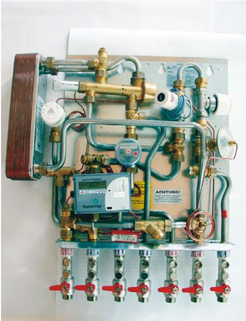
Figure 67: Apartment unit from the company Redan (picture source: AEE INTEC)
