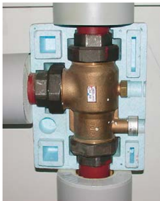
Figure 79: Admixer unit with fixed temperature adjustment without auxiliary energy (picture source: AEE INTEC).
