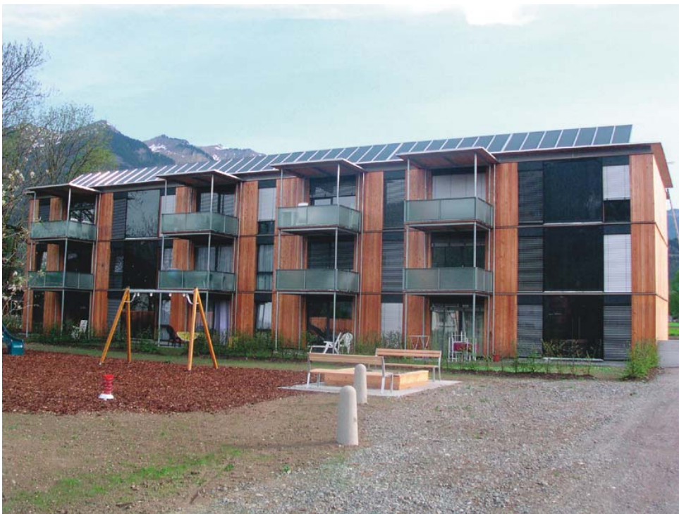
Figure 46: Modern solar-supported heat supply systems combine the hydraulic concepts with hygienic harmless in high energy efficiency (picture source: AKS DOMA, Vorarlberg, Austria).
