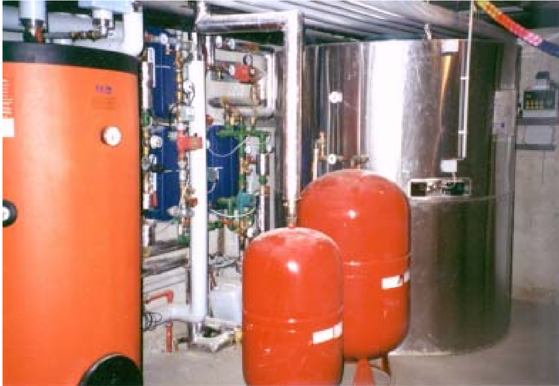
Figure 89: Two-tank system for solar-supported heating of domestic hot water and space heating based on a fore-pipe heat distribution network.
