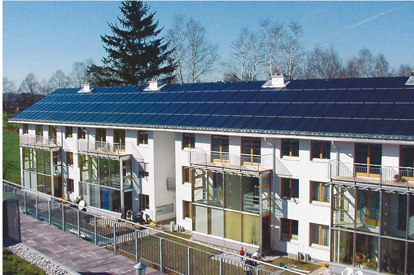
Figure 22: It is aimed to accomplish a roof consisting solely of collectors to buildings in multi-storey residential (picture source: S.O.L.I.D., Styria, Austria).
