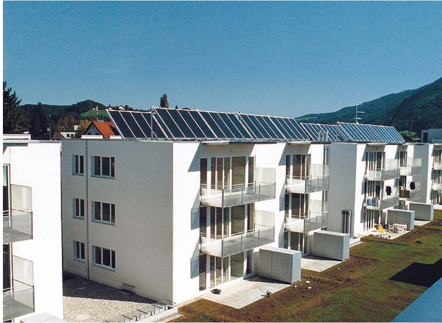
Figure 27: The entire collector area mounted on the building roof with the shortest possible way to the heating unit transfer station (picture source: Solution Solartechnik, Upper Austria, Austria).
