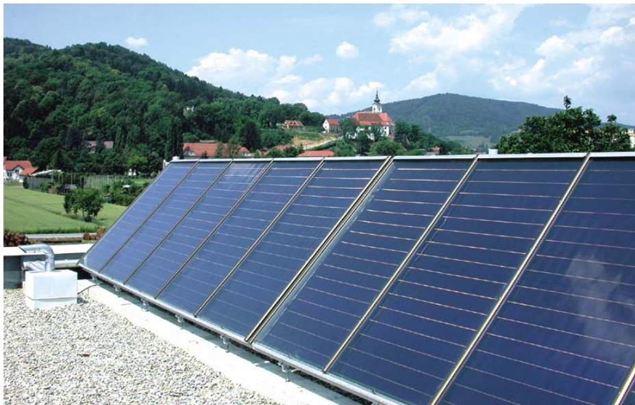
Figure 30: The collector construction is mounted on two rows of concrete foundation with a dead-load of the structure accordingly. This way the roof must not be broken through, but the static dimension of the roof has to take the weight of the concrete into account (picture source: AEE INTEC).
