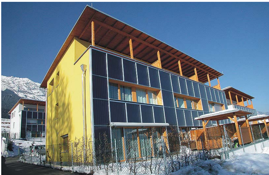
Figure 39: The effective U-value of the outer wall is reduced with the application of non back-ventilated façade collectors (picture source: SIKO Energiesysteme, Tyrol, Austria).
