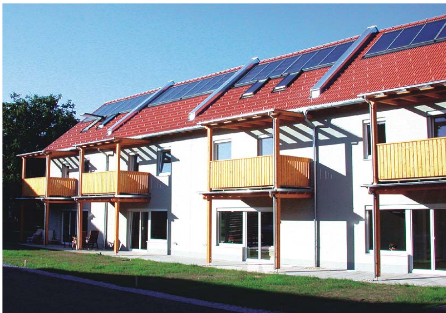
Figure 82: Solar-supported heat supply system with a decentralised domestic hot water storage tank combined with a two-pipe network (picture source: AEE INTEC).
