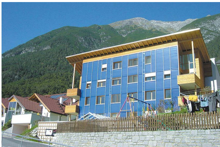
Figure 41: Application of coloured absorber layers in multi-storey residential buildings (picture source: Teufel & Schwarz, Tyrol, Austria).
