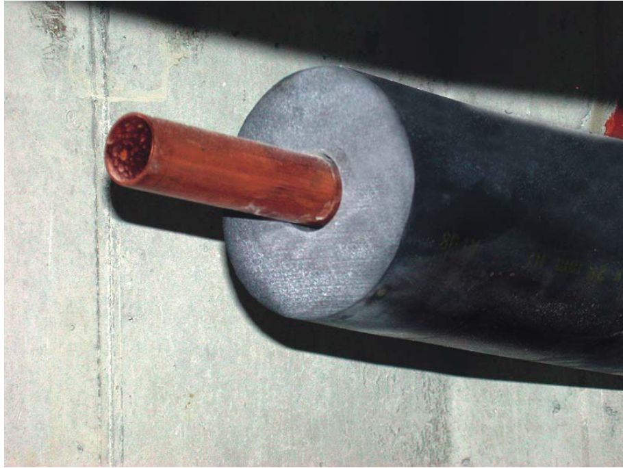
Figure 105: Pipe work for solar thermal systems, which is laid outside, should be insulated with rubber to resist temperature and water (picture source: AEE INTEC).
