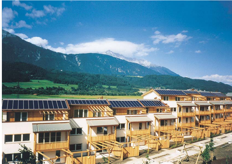
Figure 25: South orientated roof construction totally covered with collector area (picture source: Teufel & Schwarz, Tyrol, Austria).
