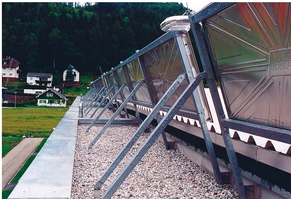
Figure 28: Each support construction break through the sealing surface of the flat roof. Because of many breakthroughs and thereby a higher risk for leakage should this mounting technique be avoided (picture source: AEE INTEC).
