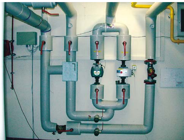
Figure 78: Parallel arrangement of the pumps for the winter use (left) and summer use (right) including an admixer unit (picture source: AEE INTEC).
