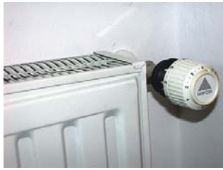
Figure 74: The room temperature is adjusted via a thermostat (picture source: AEE INTEC).
