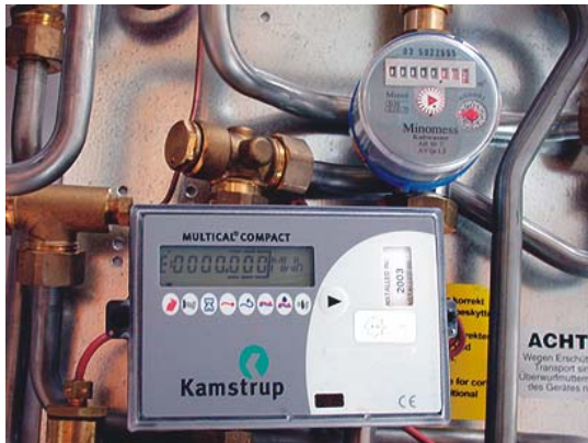
Figure 75: Arrangements of an electric heat meter and a cold water meter (example from the company Redan) (picture source: AEE INTEC).
