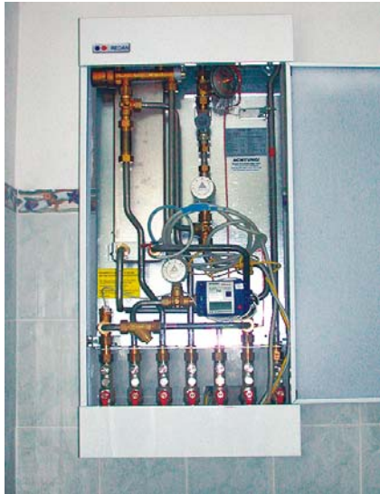
Figure 69: An on-wall apartment unit, product from Redan (picture source: AEE INTEC).
