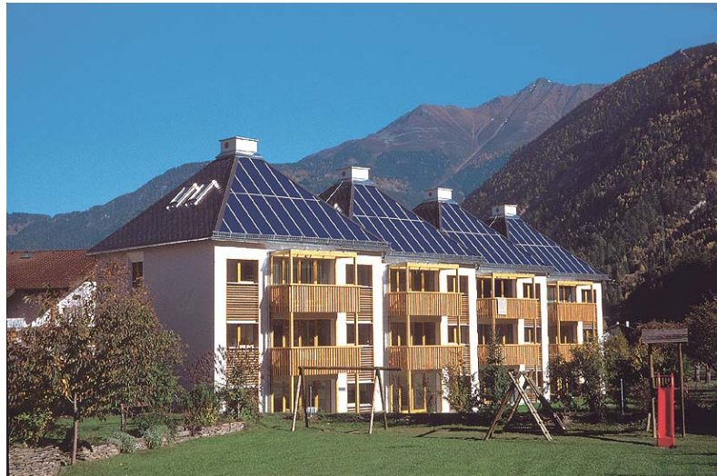
Figure 23: It is also possible to adjust the collector area to the form of the roof (picture source: Teufel & Schwarz, Tyrol, Austria).
