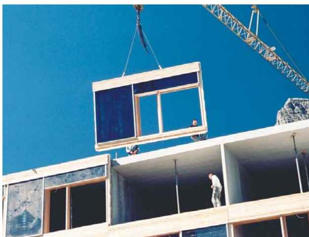
Figure 38: Mounting of a prefabricated outer wall with façade collectors without back-ventilation: the collector is not statically independent, but serves as a part of the outer wall construction (picture source: AKS DOMA Solartechnik, Vorarlberg, Austria).
