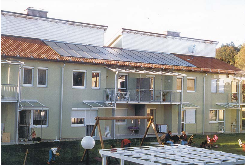
Figure 58: Solar thermal systems in multi-storey residential buildings are basically so dimensioned that no stagnation condition occurs during normal operation. However, a long period of warm weather (and thereby a charged energy storage tank), an electrical power outage or a technical defect could just as well cause this condition (picture source: AEE INTEC).
