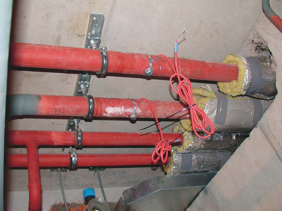
Figure 107: No reduction or even discontinuity of insulation by penetrations in walls or ceilings.
