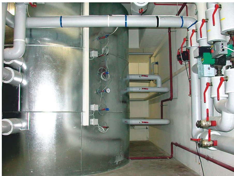
Figure 102: Single-storage-unit systems with thoroughly performed heat insulation reduce the heat losses drastically.
