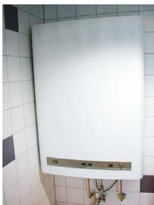
Figure 83: A decentralised domestic hot water storage tank with a two-pipe network. Neither volume nor the arrangement differs from a conventional off-peak energy storage unit (picture source: AEE INTEC).
