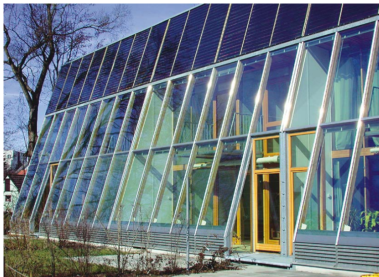
Figure 24: Solar collectors can be adjusted to existing geometrical building constructions (picture source: AEE INTEC).
