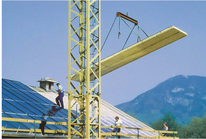
Figure 20: Crain assembly of large-area collectors (picture source: S.O.L.I.D., Styria, Austria).
