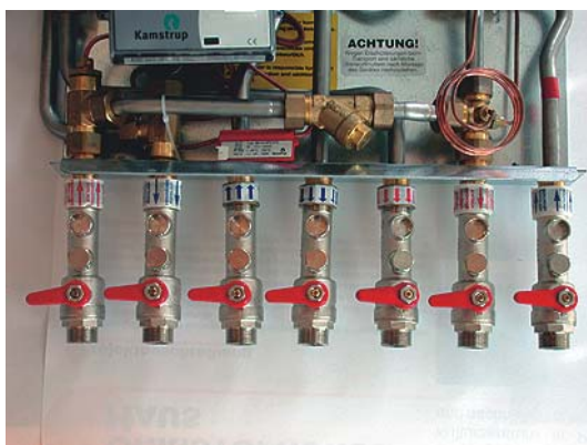
Figure 76: The central arrangement for the shut-off valve enables a quick act in case of emergency or for maintenance (example from the company Redan) (picture source: AEE INTEC).
