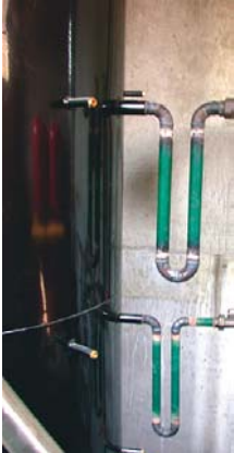
Figure 100: Thermosiphon connections in the installation practice (picture source: AEE INTEC).
