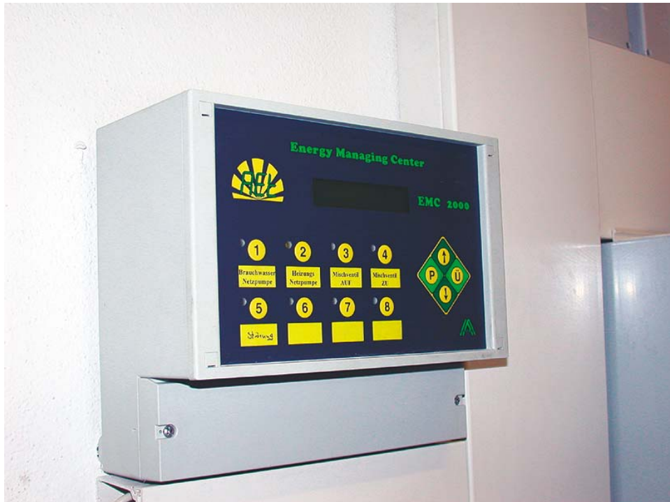
Figure 114: Exemplary demonstration of a central regulation device with an integrated data logger and remote control monitoring.
