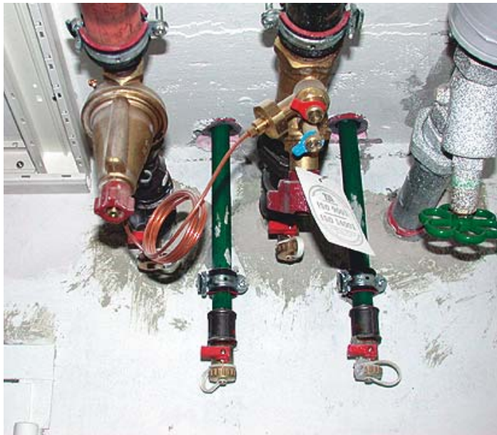
Figure 77: Riser strings adjusted through the differential pressure regulation. Detail: Riser strings can easily be bled through a maintenance friendly positioning in the basement.
