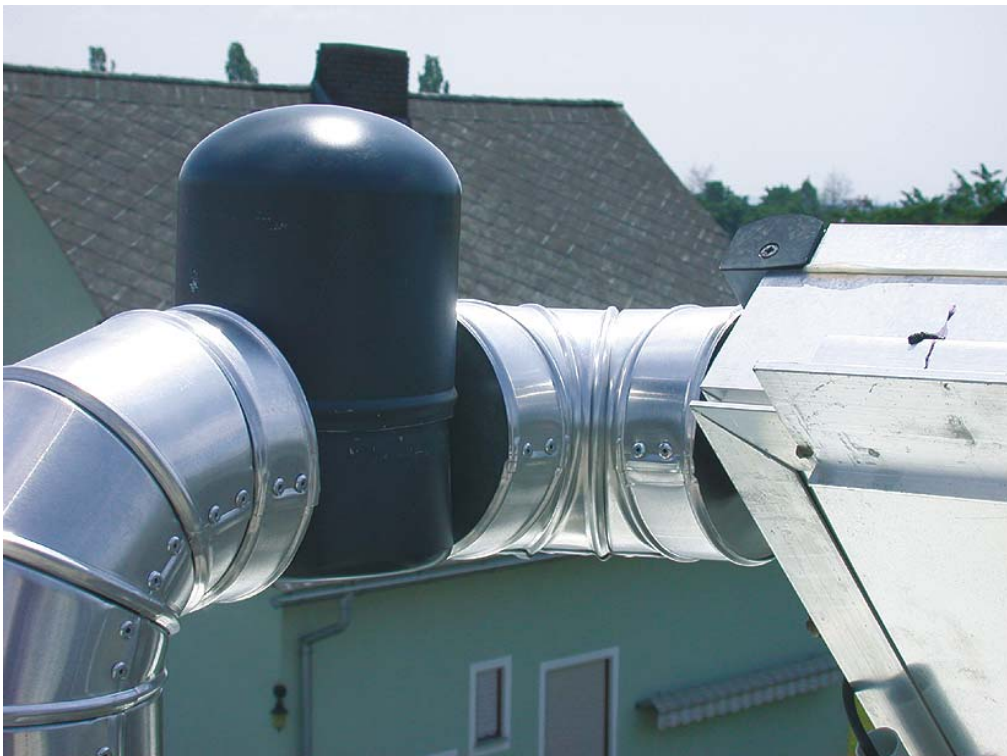
Figure 57: Configuration of a temperature resistant, manual bleed points with weather-protection and heat-insulation (picture source: AEE INTEC).
