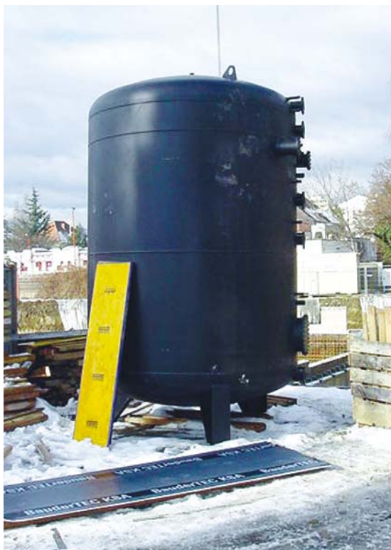
Figure 42: Energy storage tanks in multi-storey residential buildings have already to be integrated in the planning phase due to their size and position (picture source: AEE INTEC).
