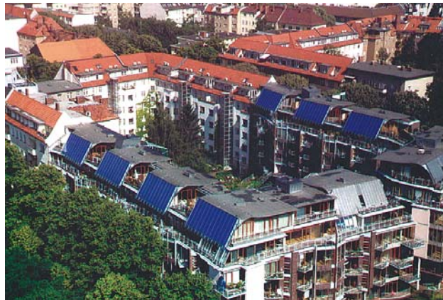
Figure 3: 274 m 2 solar thermal collector area produced by an Austrian manufacturer on a housing estate with 197 apartments (picture source: Kappei SOLAR FUTURE TECHNIK, Germany).
