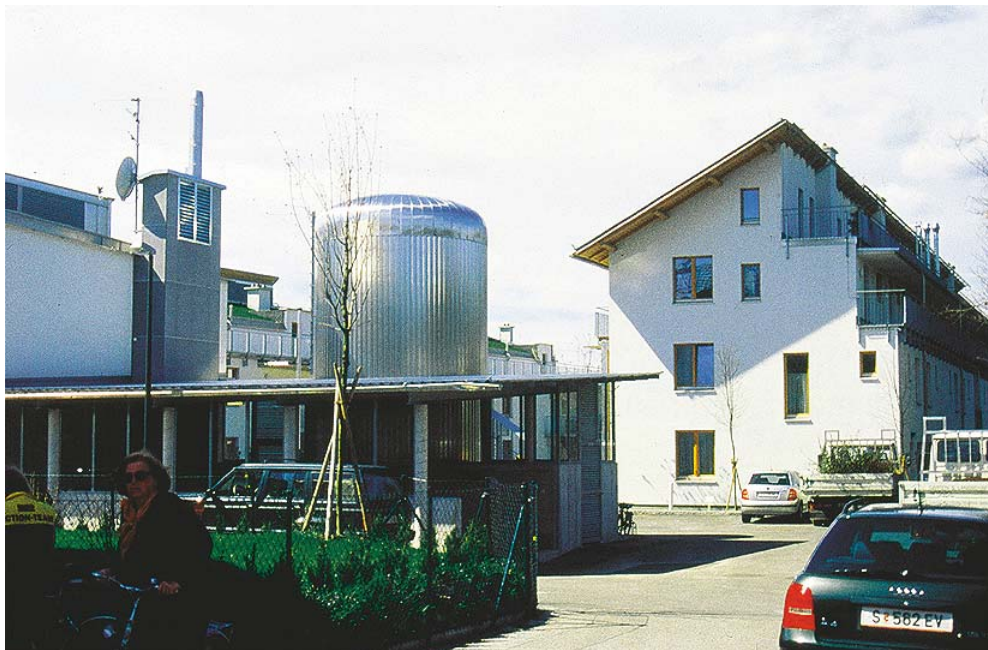
Figure 45: Part of the 100 m 3 energy storage tank appears from the underground in the middle of the housing estate Gneis-Moos (picture source: AEE INTEC).
