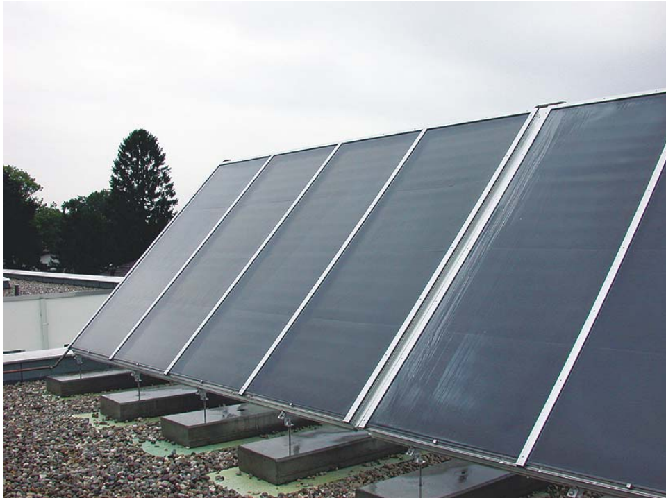
Figure 31: The collector construction is mounted on diagonal arranged concrete foundations with a dead-load of the structure accordingly. This way the roof must not be broken through, but the static dimension of the roof has to take the weight of the concrete into account (picture source: AEE INTEC).
