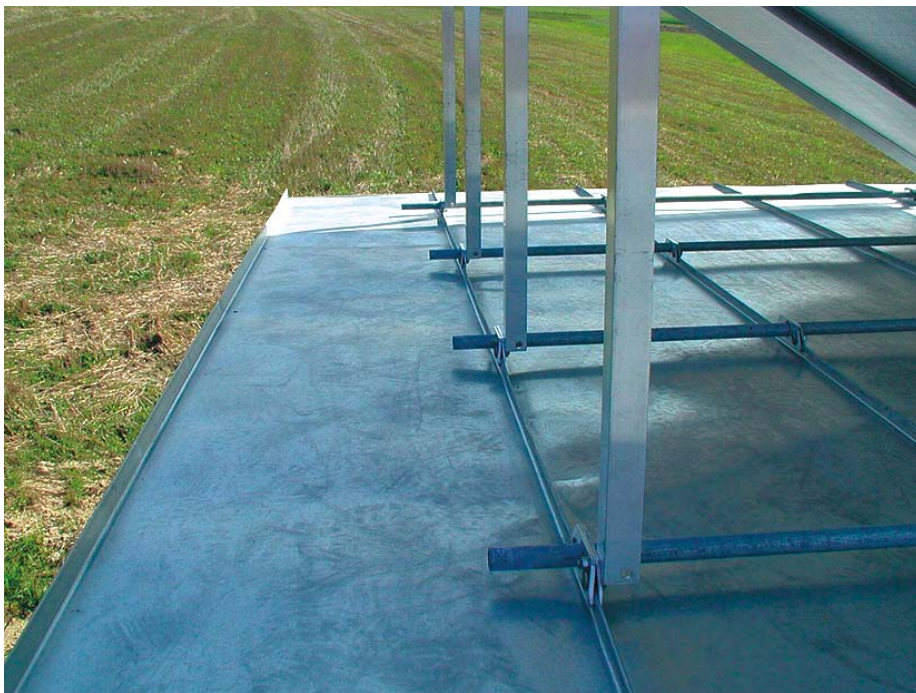
Figure 32: Clamping profiles mount the collector frame to the standing seam (picture source: Solution Solartechnik, Upper Austria, Austria).
