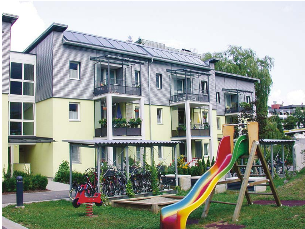
Figure 48: Solar thermal system in a multi-storey residential building should be operated through the low-flow principle (picture source: AEE INTEC).
