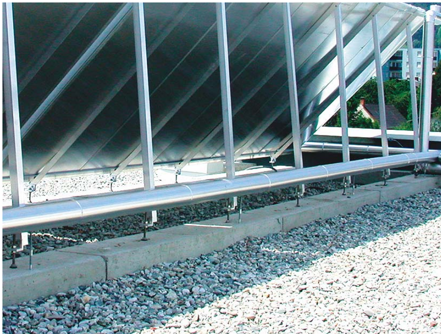
Figure 106: The rubber surface of the piping coat should constantly be protected against UV-light and damage from animals through a sheet-metal jacket (picture source: AEE INTEC).
