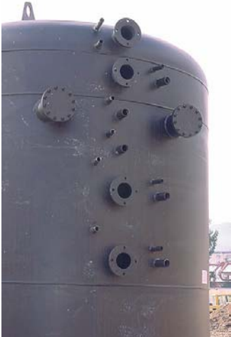
Figure 64: The heat storage tank acts like a hydraulic switch between the heat supplier and consumer. The properly arranged connections and sensor devices to the storage tank have to be fixed in detail at the planning state (picture source: AEE INTEC).
