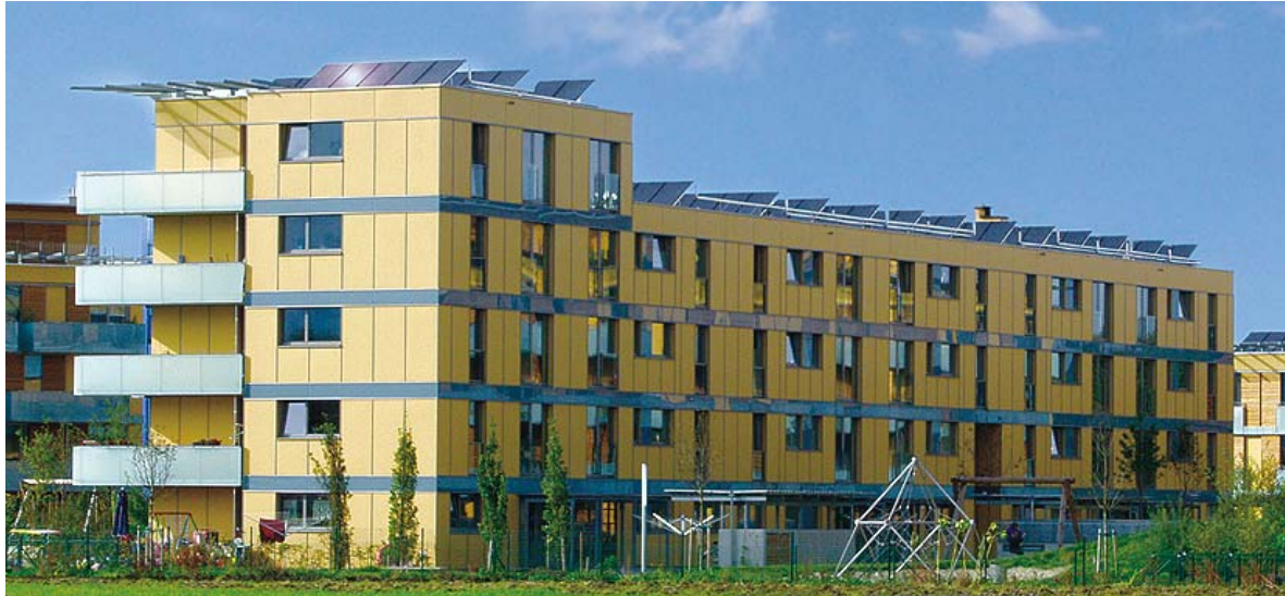
Figure 66: Solar-supported heat supply through a two-pipe network with apartment units in the housing estate "Stieglgründe" in Salzburg, Austria (picture source: Sonnenkraft, Carinthia, Austria)
